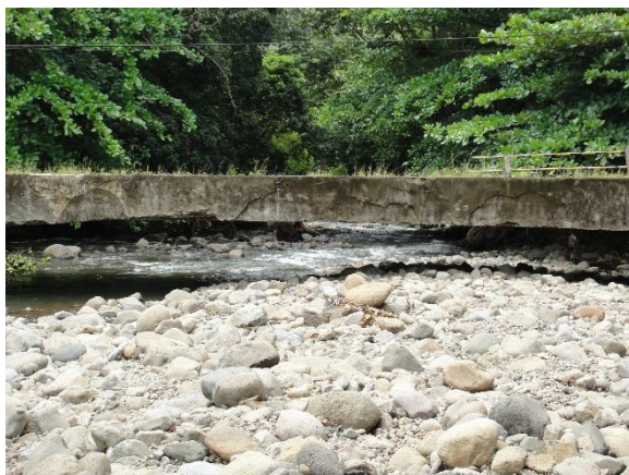
Figure 10 – Heavily silted river channel
