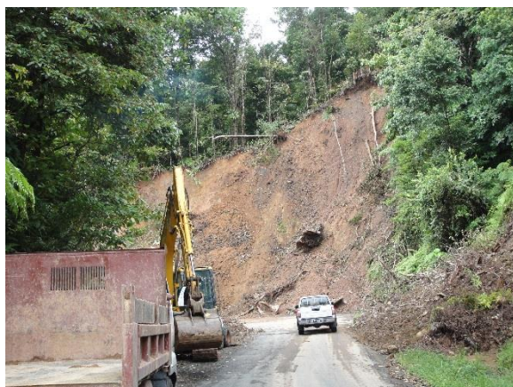
Figure 5 – Landslide being cleared
