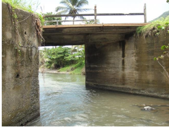
Figure 16 – Small bridge at San Sauveur near shoreline
