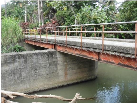
Figure 18 – Hatton Garden Bridge at chainage 20km
