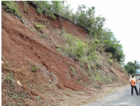
Figure 14 – Unstable slopes after landslide at Castle Bruce
