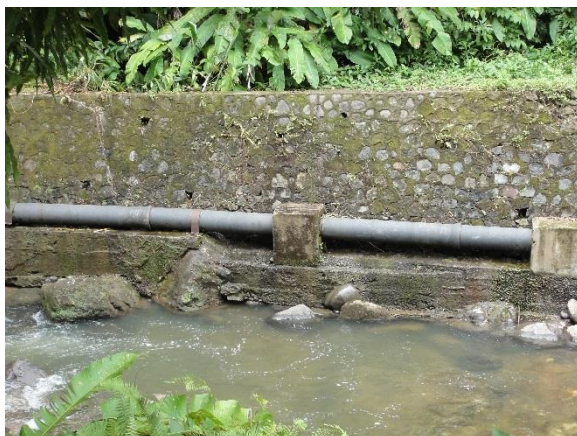
Figure 8 – Scour to bridge abutments due to high flows of river
