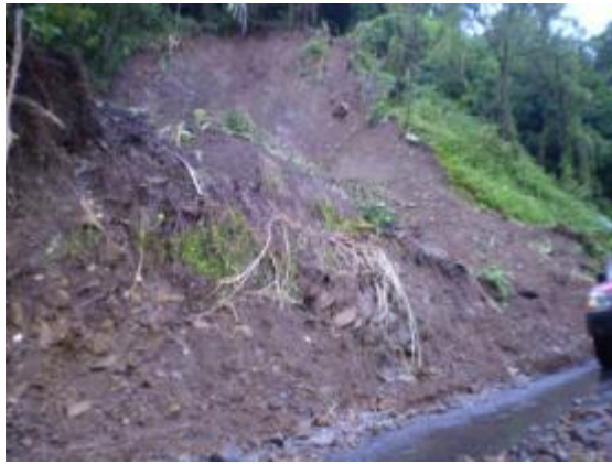
Figure 15: Land Slippage at Petite Souffriere.
