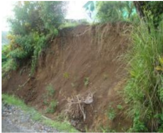
Figure 1: First Landslide on Jalousie Road
