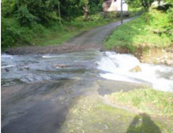
Figure 9: Flooding of crossing within Castle Bruce Village
