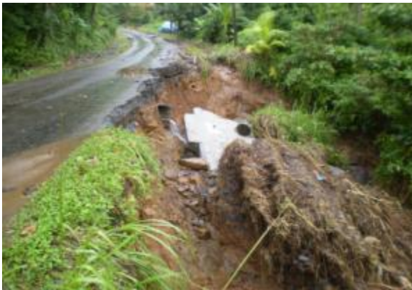
Figure 11: Road edge and drainage failure at San Sauveur
