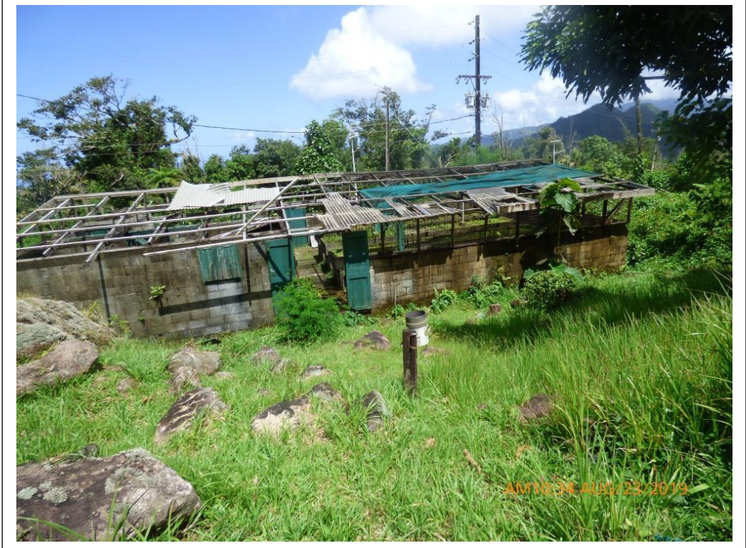
Photo: Propagation Building to be rehabilitated and upgraded
