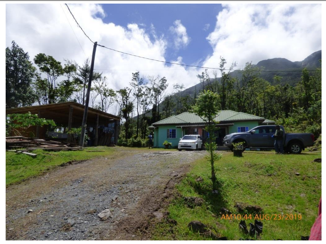
Photo: Caretaker's House (green) and Drying Shed
