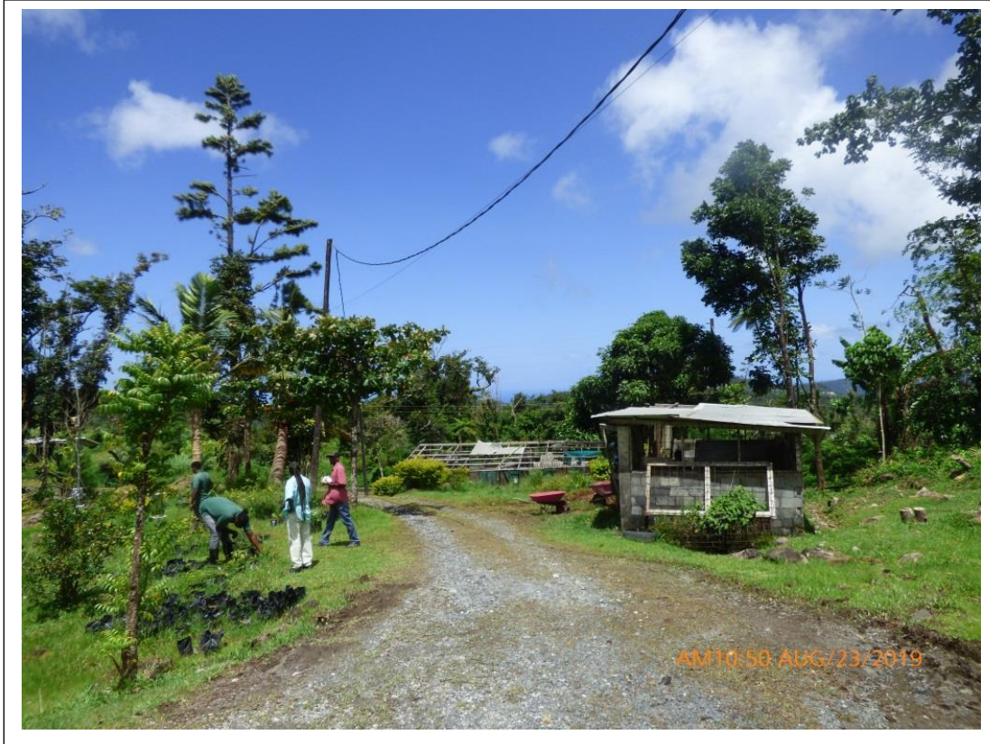
Photo: View of site (some buildings to be partially or fully demolished)
