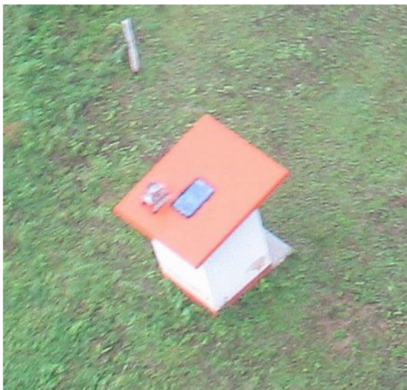
Figure 15: Instrument shelter constructed in 2010 by Autoridad del Canal de Panama (ACP) with embedded solar panel and rain gauge funnel on the precast concrete roof. Photographed from heliconter.
